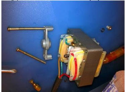
On the upper side of the motor spindle a small clear plastic washer fits tightly on the motor spindle. I slid this off and stored safely.
