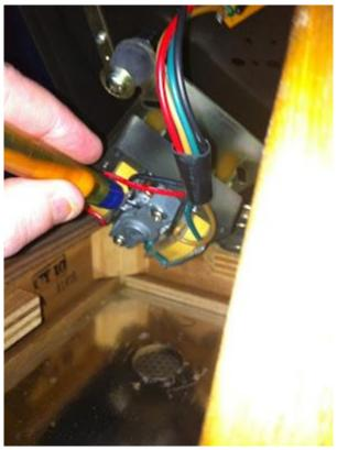
Again I used my precision oiler. Gently probing with the nozzle while lifting the motor pulley from above to create a gap where the oiler might find the lower part of the motor spindle.
